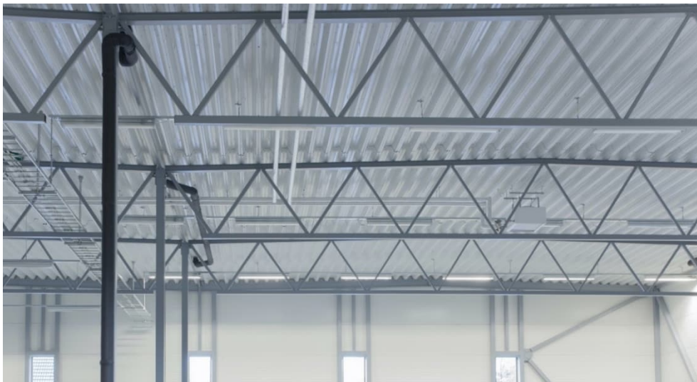
Fig. 4.23 Example of roof system with deep decking [31]
