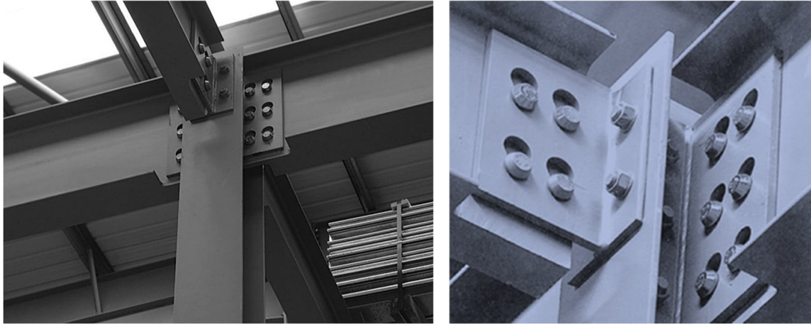
Fig. 4.16 Quicon connections [34]
