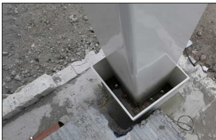
Fig. 4.9 Example of accessible base connection [30]
