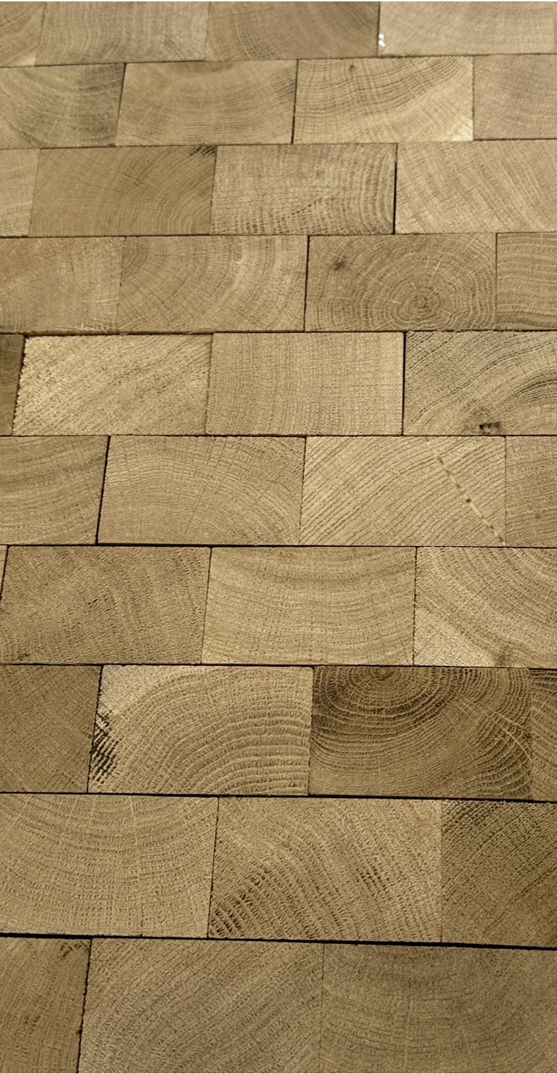
Kubbegulv i bue
